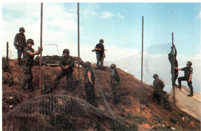
Marines erecting a fence at their Beirut compound this month to deflect bomb fragments
